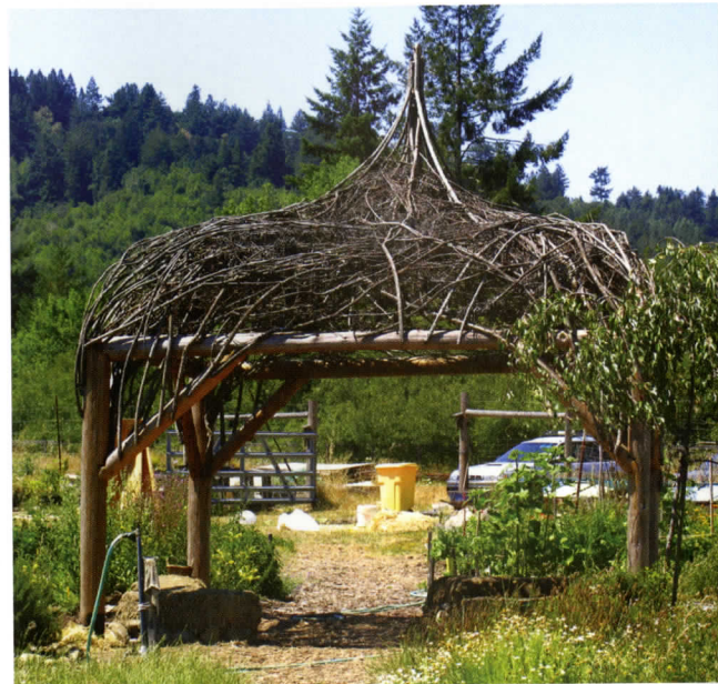
FIGURE 13.38 This graceful domed gazebo inside the garden at Salmon Creek School shelters a ring of cob benches. Handcrafted by a local artist, the shade structure is supported by sturdy logs harvested from the school site. Its peaked top is woven from a collection of artfully arranged branches shaped to form a distinctive rounded roof with a pointed top. 10
