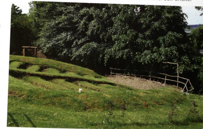
FIGURE 13.6 This amphitheater at Ebchester Church of England School in Great Britain was carved directly into the hillside. The seats are planted with grass and the space between the tiers is the natural soil onsite.
