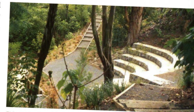
FIGURE 13.5 This beautiful forest amphitheater at Meadowbank School in New Zealand takes advantage of a natural hillside and its inviting shady setting. 2
