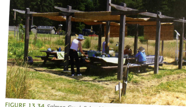
FIGURE 13.34 Salmon Creek School has a large seating area with four picnic tables, sheltered by a permanent structure of heavy wooden beams. During warm spring and fall weather, the school hangs temporary bamboo screens on top of the canopy to cool the classroom space below.
