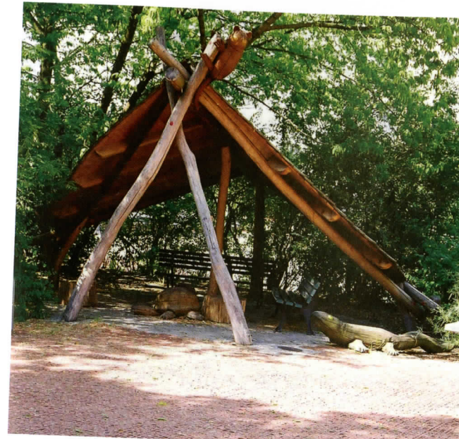
FIGURE 13.40 This handcrafted, artful shelter on the grounds of Peter Joseph Lenné School in Germany has a peaked roof that protects several seats and benches. 11
