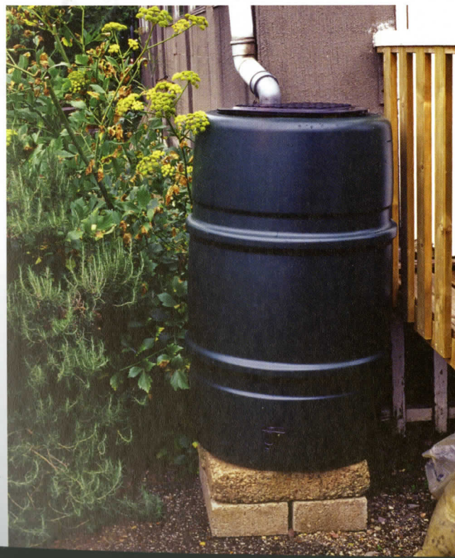
FIGURE 5.19 Cowick First School in southwest England teaches its young students that water is a precious resource. This concept is noted on schoolyard signs and reinforced at the school with the use of low-flow bathroom sinks and toilets. A rain barrel also collects stormwater runoff from the school's roof for watering the garden. 19
