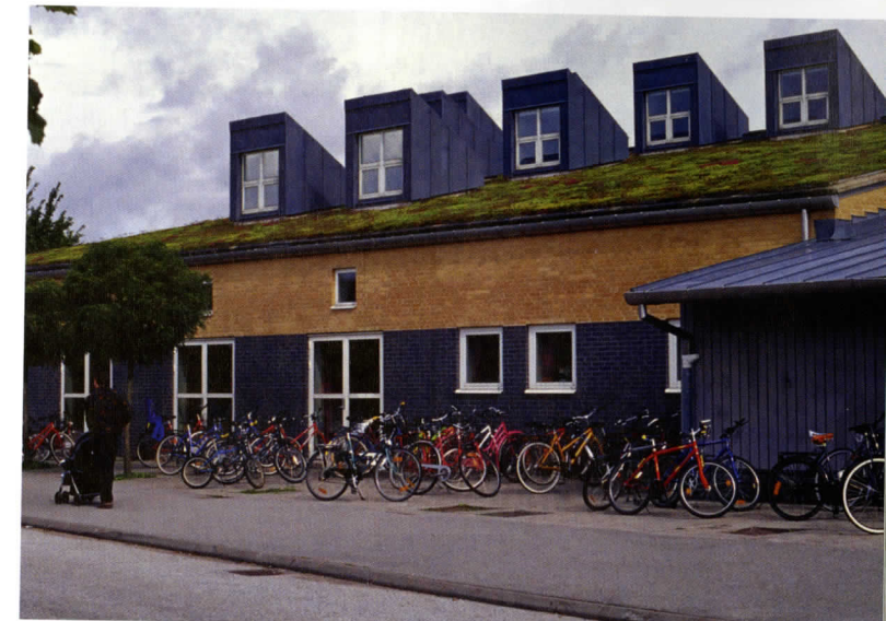
FIGURE 5.16 The living roof at Gunnesbo School in southern Sweden is planted with drought tolerant, waxy-coated sedums that are well-suited to hot, dry roof conditions.
