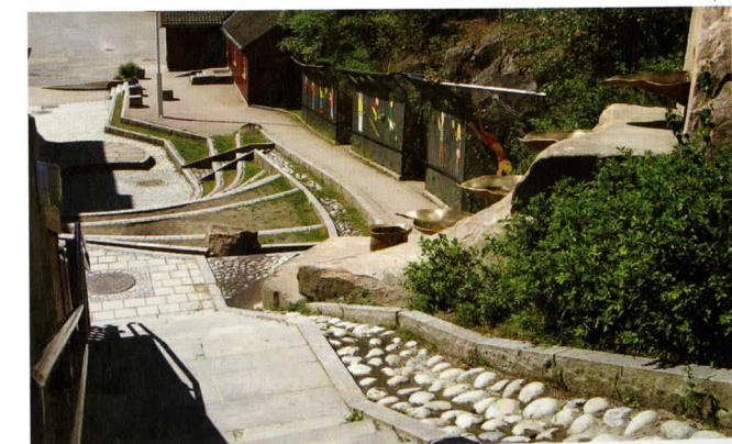
FIGURE 5.9 The cobblestone runnel at Svendstuen School in Oslo, Norway, directs stormwater as it flows downhill and keeps the stairs free of puddles.
