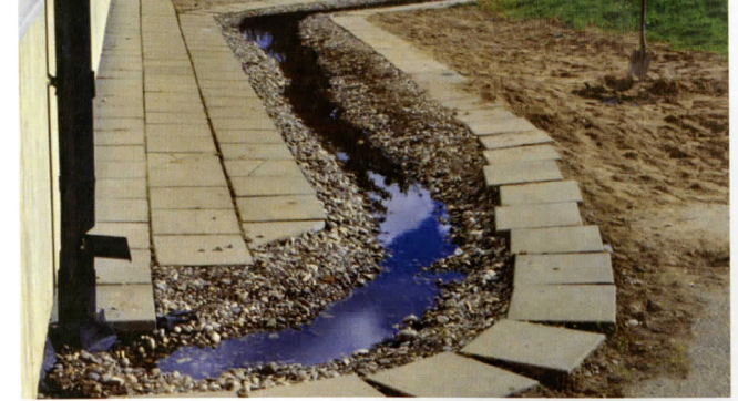
FIGURE 5.7 Mårten School in southern Sweden has a small pond fed by runoff from the school's roof. The stormwater flows across the roof, down the building's downspout, and through a long winding channel at ground level before filling the pond. 9
