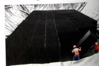
FIGURE 5.25–5.27 Open Charter Elementary shown before and after schoolyard renovation. Underground cistern during construction (below).
