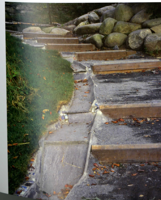
FIGURE 5.8 Playful drainage system at Bergen Steiner School.
