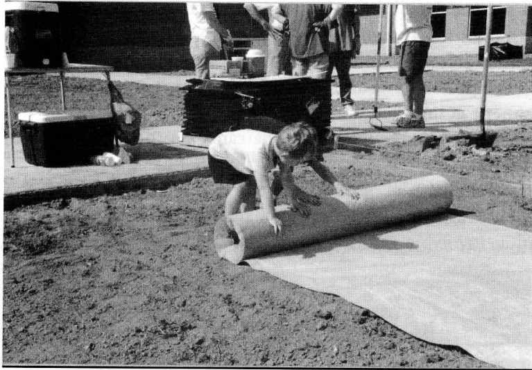
FIG 2-34. This child helps roll out fabric in preparation for the playground safety surfacing material. (COURTESY OF GINA K. MCLELLAN.)
