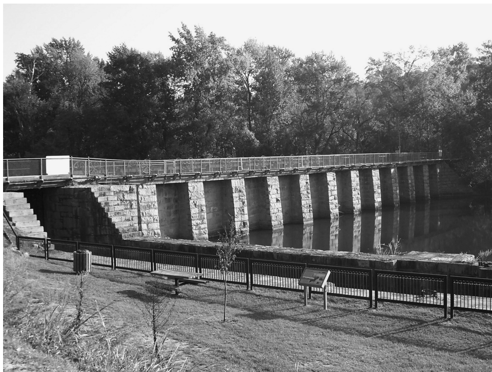
Figure 2. Historical dam and canal structure dating to the 19th century, located on the Three Rivers Greenway.
