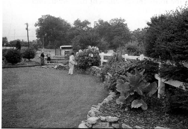
FIG 5-20. This retaining wall at Wonderland Gardens, GA is made from a combination of recycled concrete sidewalks and stone. (COURTESY OF MARY TAYLOR HAQUE.)
