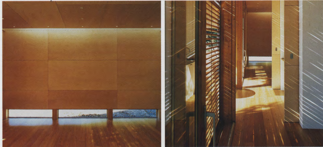
The basic concept of the project and its elemental geometry made it possible to use traditional wood construction techniques. The openings are carefully designed to provide adequate lighting, according to need, or to highlight certain aspects of the setting.
