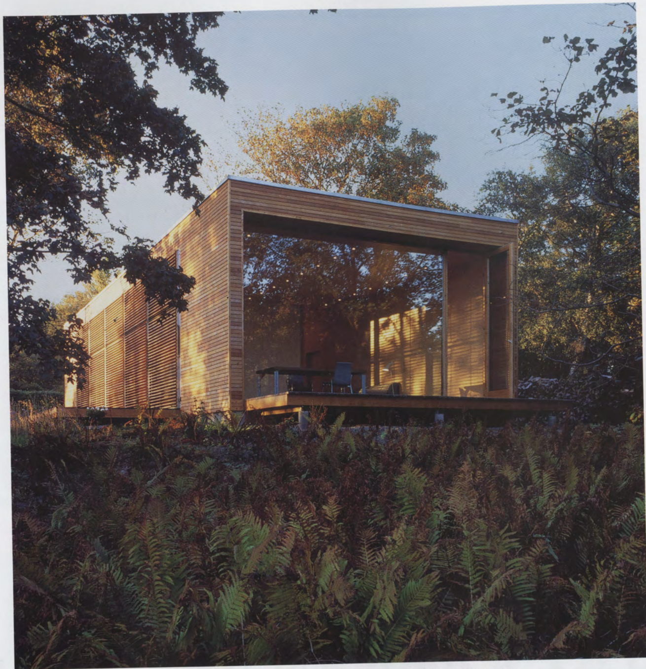
The wooden decks enhance the image of the house as an object floating above the dense growth of ferns covering the site.
