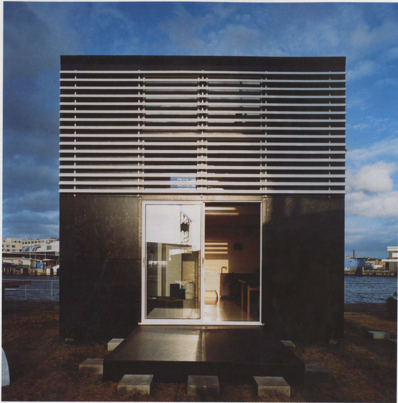
The platform at the entrance and the blinds on the upper level can be adjusted in accordance with how the building is being used or the amount of light desired.
