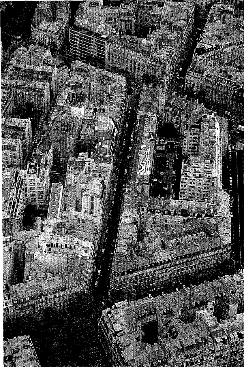
FIGURE 4.19 Perimeter blocks in central Paris, France. Perimeter block development has a number of advantageous characteristics/features: explicit public and private sides; the capacity to accommodate different densities of development; and a public façade that both physically defines and 'socially' addresses an urban space
