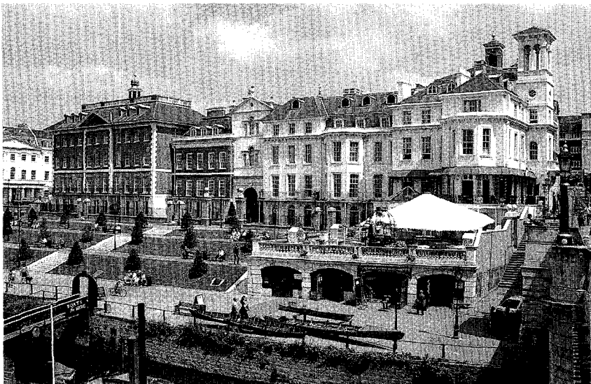
FIGURE 7.20 Richmond Riverside, London. Although the façade suggests a number of separate buildings, this development actually consists of a few large office buildings with open office floors extending across what we are led to assume are party walls
